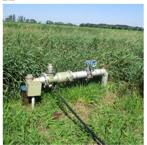
"This chemigation system is permitted by the Minnesota Department of Agriculture (MDA) to inject liquid fertilizer and has the required operational anti-pollution device back-check valve, a low pressure drain and vacuum relief. The hose attached to the low pressure drain directs any chemigation water away from the well that may get behind the back-check valve when the irrigation system is shutdown."
